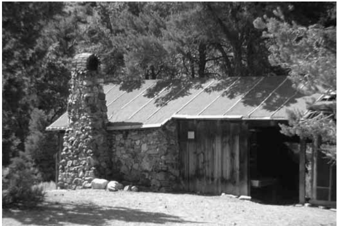
FIGURE 20. Charles Camp's cabin at his ichthyosaur dig near the ghost town of Berlin, Nevada. Camp constructed his cabin from lumber borrowed from some of the buildings in Berlin and at Union, another ghost town also nearby. Camp and Welles and their assistants and students used this cabin from 1955 to the 1960's for living, laboratory work, storage, and packing fossils. Photograph by J.H. Lipps, 1994.
